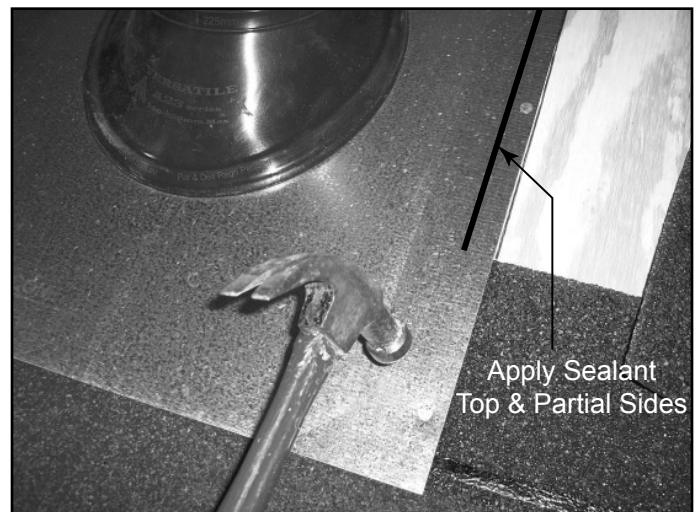
Figure 10.13 Slide Flashing Down, Secure & Apply Sealant
