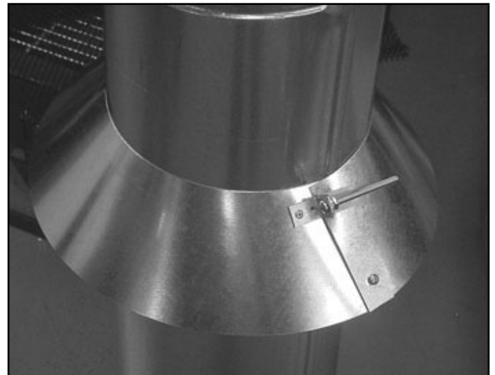
Figure 10.16 Assembling the Storm Collar Around the Pipe
