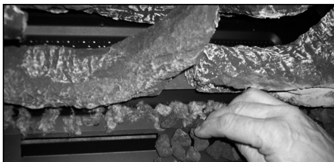
Figure 14.5 Placement of Lava Rock
