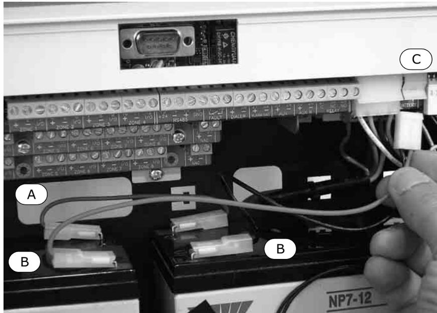
**Figure 39 - Connecting the batteries**
