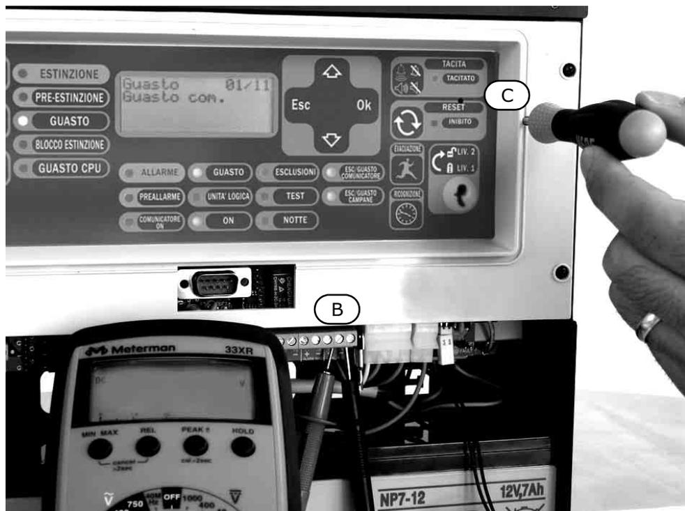
**Figure 34 - Adjusting the voltage charge**
