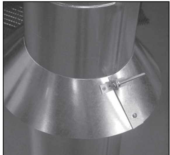
Figure 2.22 Assembling the Storm Collar Around the Pipe
