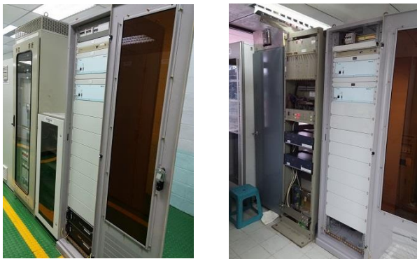
Fig. 9 (Left) Teleprotection cabinet installed at ABCD and (Right) Teleprotection cabinet installed at EGAT-RY1 substation
