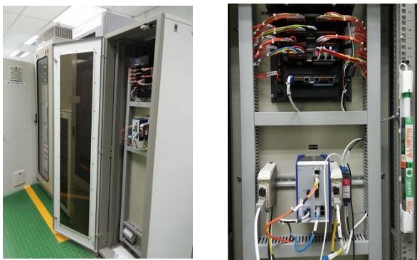
Fig. 10 RTU cabinet installed at ABCD Power Plant
