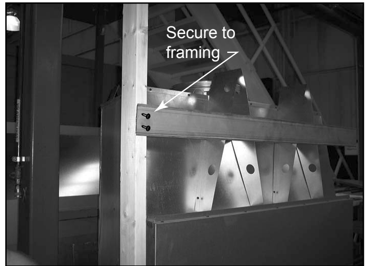
Figure 12.14 Secure to Framing
