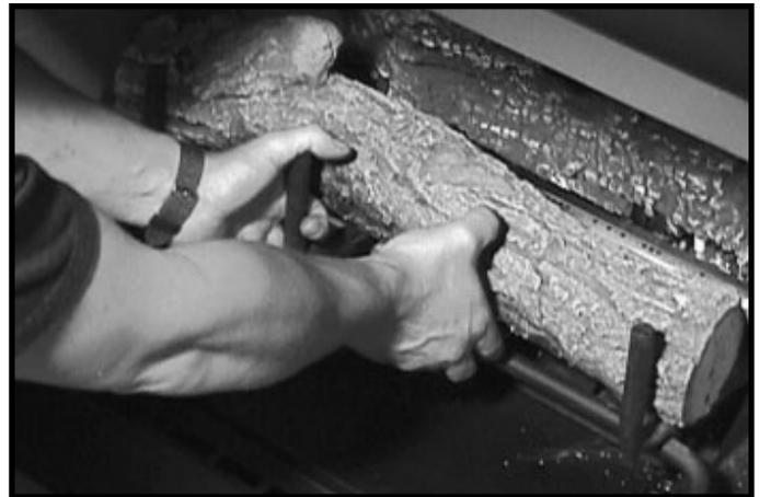
Figure 14.7 Remove Grate/Log Assy.
