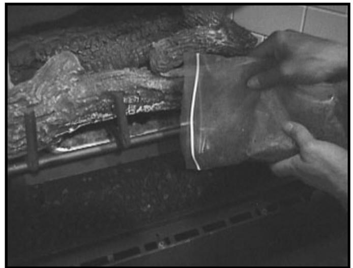
Figure 14.3 Placing the Lava Rock
