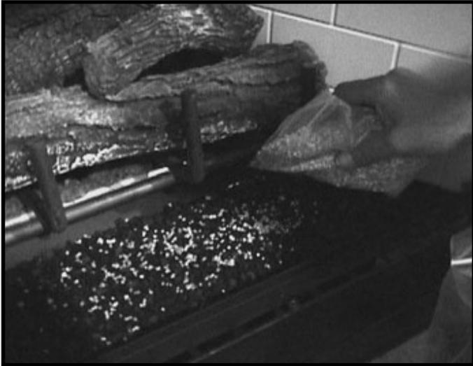
Figure 14.4 Placing the Vermiculite
