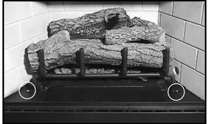
Figure 14.6 Remove Two Screws Holding Front Grate/Log Assy.
