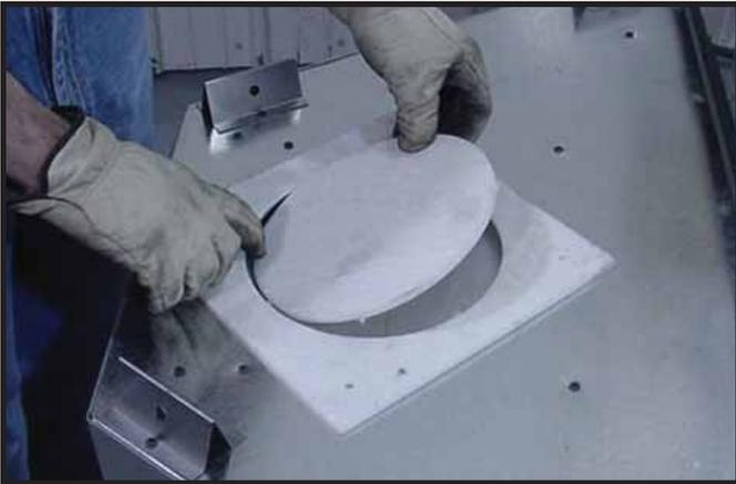
**Figure 9.2** Remove the center insulation plug.
