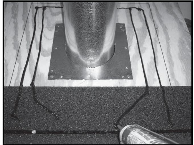
Figure 10.20 Apply Sealant
