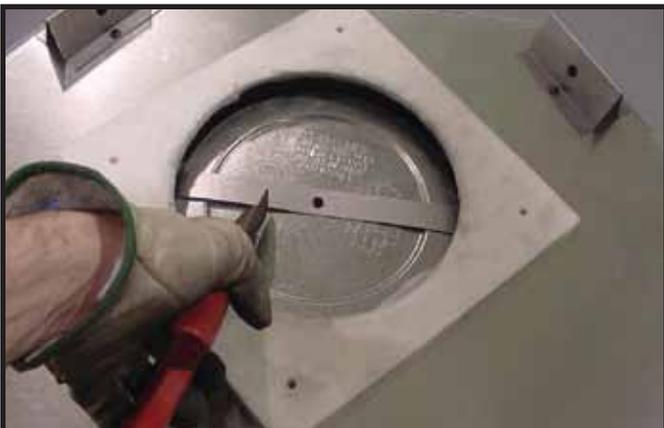
**Figure 9.3** Cut the metal retaining band and fold the sides out.
