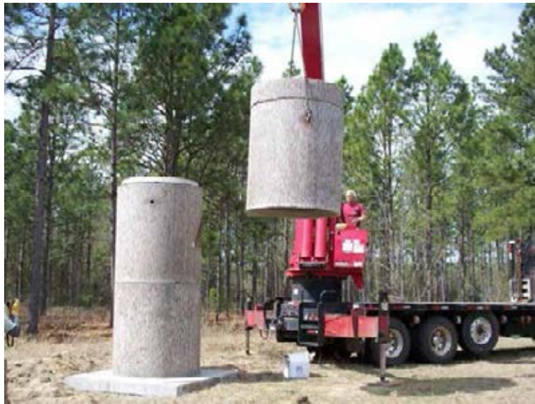
Figure 19. Construction of an artificial bat roost.
