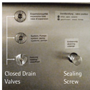
Figure 3-2: HTF Drain Valves and Sealing Screw
