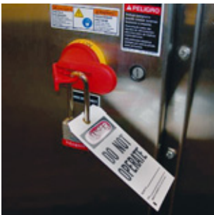
Figure 11-3: Lock Example for FT16 Power Disconnect
