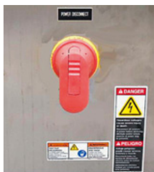
Figure 3-1: Power Disconnect Switch in ON Position
