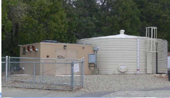
Dobbins Fire Water Tank and Pump House
