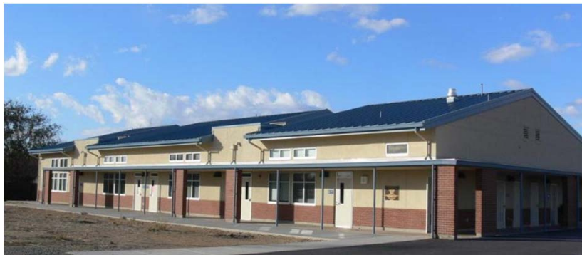
Johnson Park Classroom Building
