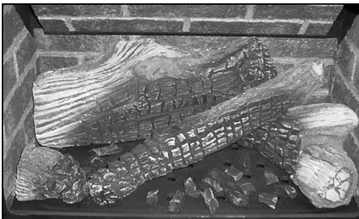
Figure 59: Log Placement with Rock Wool.
