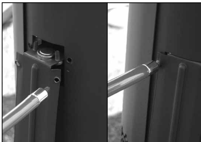
Figure 49: Spill switch installation.
