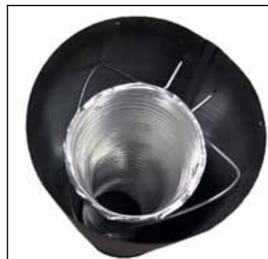
Figure 20: Wire Spacer in Place.
