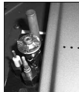
Figure 13. Ignitor assembly beside the burner.
