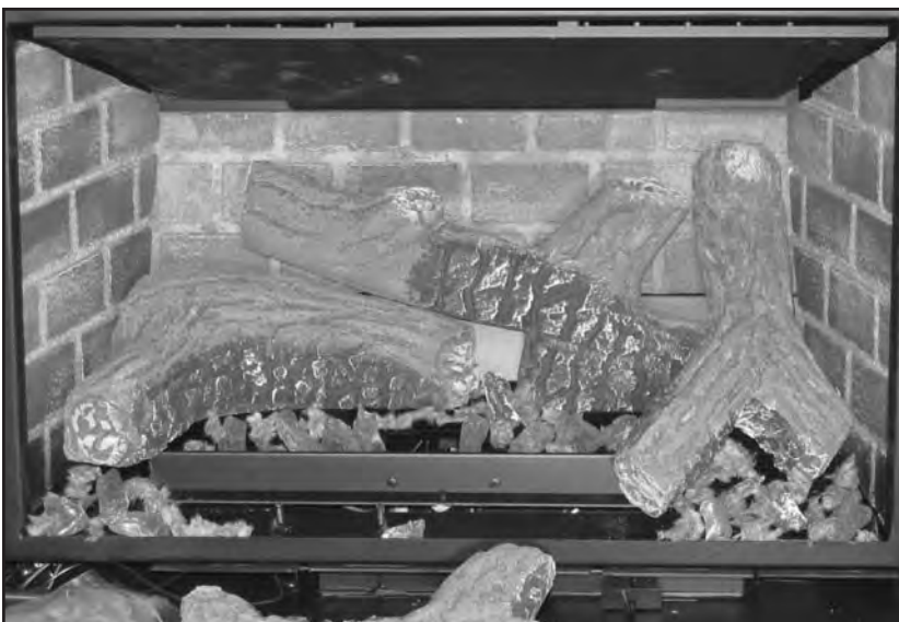
Figure 77. Fifth Stage Log Set Installation.
