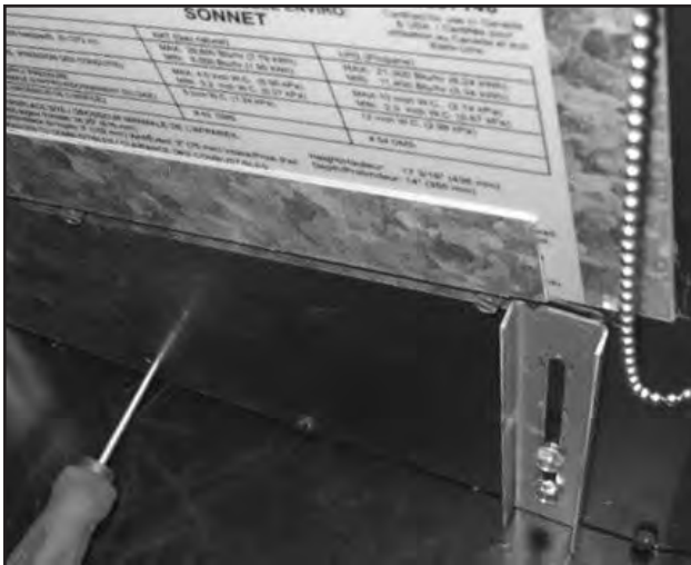
Figure 15: Resetting Receiver from Outside.
