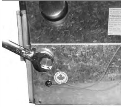
Figure 27: Remove Brass Cap.
