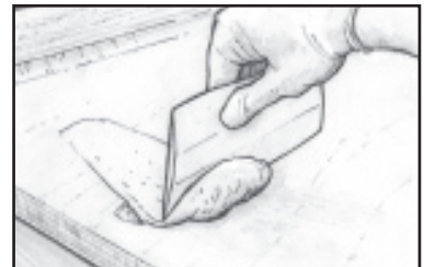
Trowel epoxy mixed with 407 Low density Filler to peanut butter Consistency into voids.
