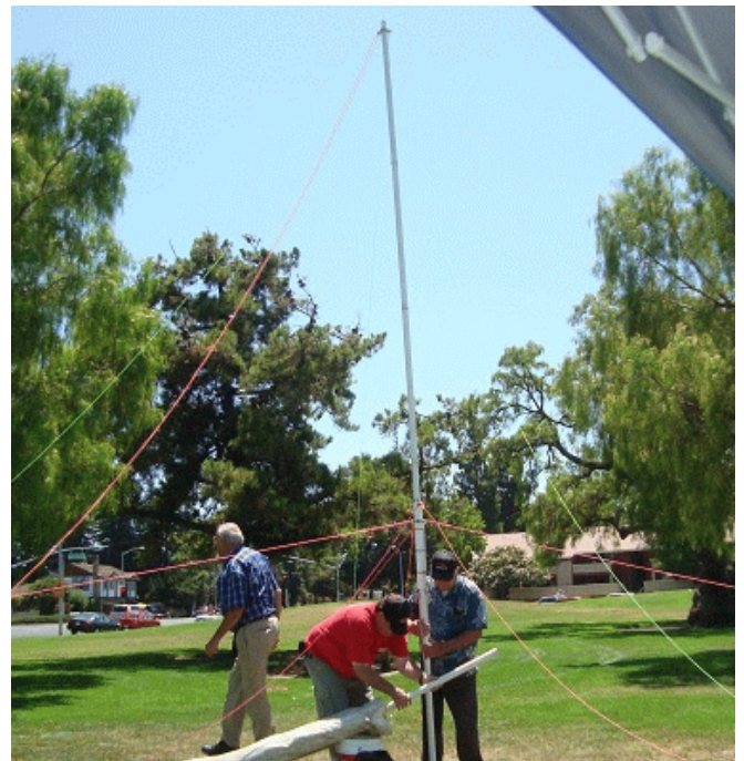
Lou (right) lifts the stack while Gregg (red shirt) slides the next 4-ft section under the PVC water pipe which stabilizes the stack.
