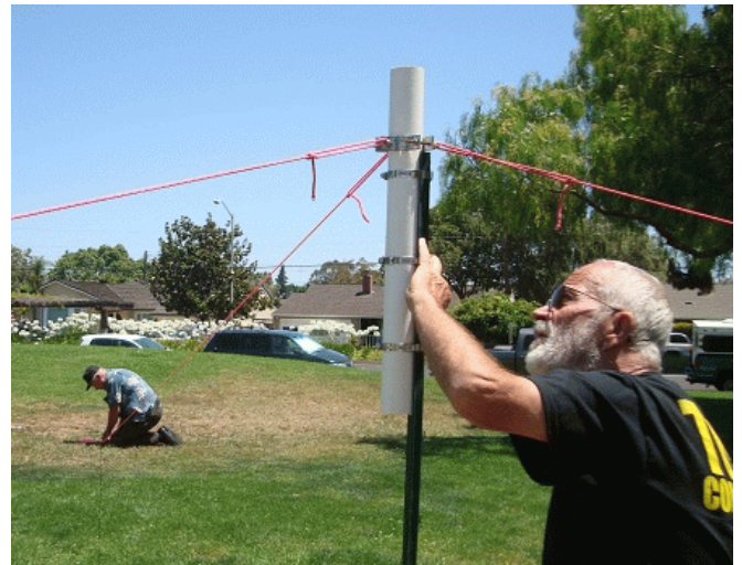
The secret to pushing up 4-ft x 2-in sections of fiberglass mast. The bottom of the 2 1/8" I.D. white PVC water pipe that John is looking at is held 4-ft 6-in above the ground by the fencepost. Lou stakes a guy line center left.
