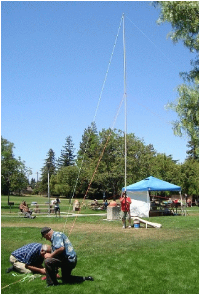
Gregg braces the base of the mast at max height of around 36.5 feet, while Goetz and Lou stake.
