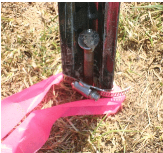
Stake and radiator clamp anchoring the fencepost.
