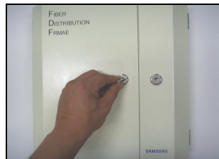
18. Finishing the Termination Box
