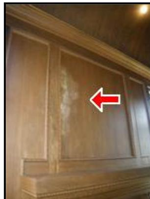
🔧 (3) There is a moisture stain on the 2nd level den wall, which you should ask the sellers to explain or have explored further. The stain was dry at the time of the inspection. We could not confirm that repairs have been
