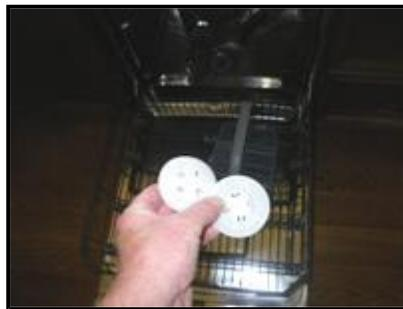
**9.1** The garbage disposal needs a new throat insert, which is a simple installation that typically does not require dismantling the unit. Note: the insert was observed in a kitchen drawer.
