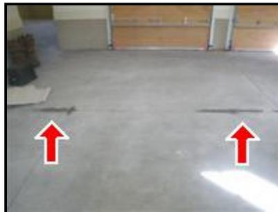
(2) No expansion joint was provided for the garage floor at the perimeter of the slab. Cracking of the garage slab or adjacent foundation wall may occur. Note that this is a common defect and the addition of an expansion joint would be an expensive repair.
