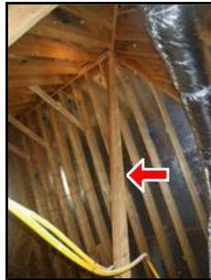
🔧 (3) At the front of the home, the very peak, there is a possible roof leak. We observed roof sheathing that was lightly stained. The stains may only be sap, but they more closely resemble water stains. We recommend an evaluation by a competent roofing contractor and/or observation during a period of heavy or prolonged rain.
