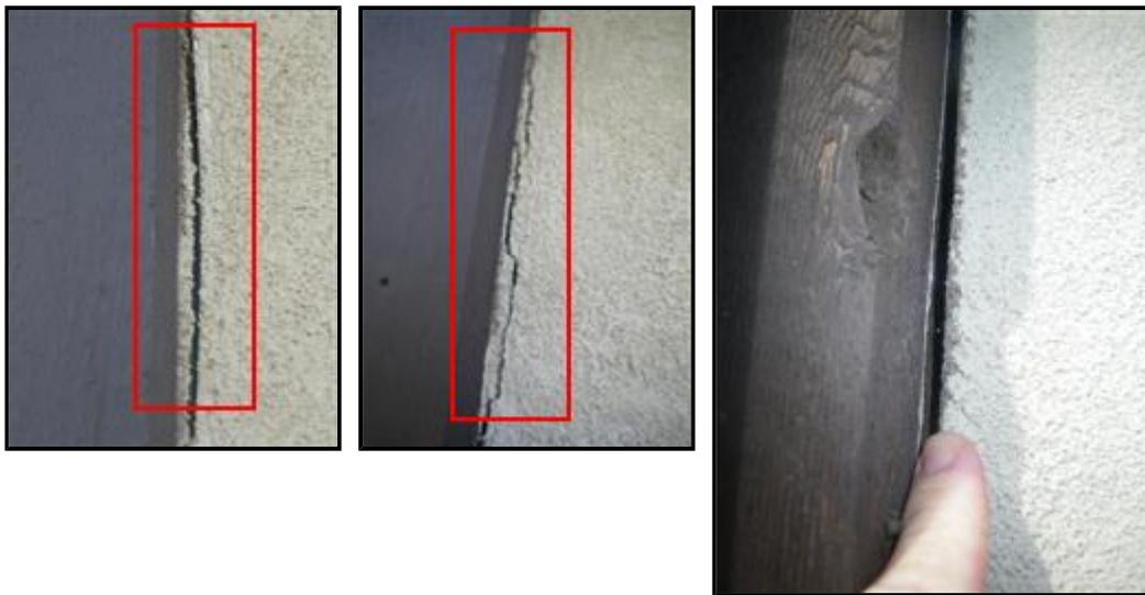
(4) There are large gaps at various locations where different wall materials meet. The wall structure and insulation was visible. Sealing the gaps to prevent water entry and structural damage is recommended. *Note that we did not inspect behind the wall cladding and there is a possibility that structural damage may already exist to some degree.*
