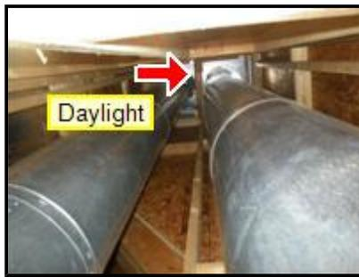
**3.3** The roof includes one or more skylights, which are notoriously problematic and a common point of leaks. There are different methods of installing them and, although opinions will vary, some methods are better than others. Therefore, it will be important to keep the area around them clean and to monitor them for evidence of leaks.
