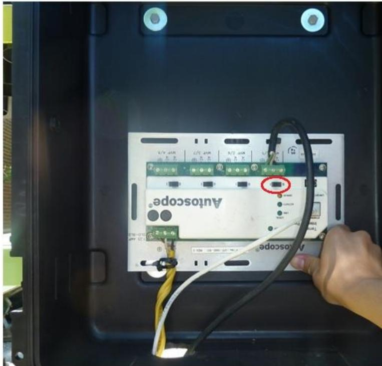
3. Make sure that the switch (marked RED) near to the black camera cable is in the ON position. If it is not, then the camera will not be powered.
