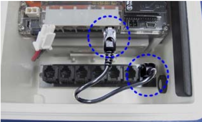
Installing expander cable
