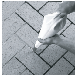
Figure 23 - Grouting Brick
