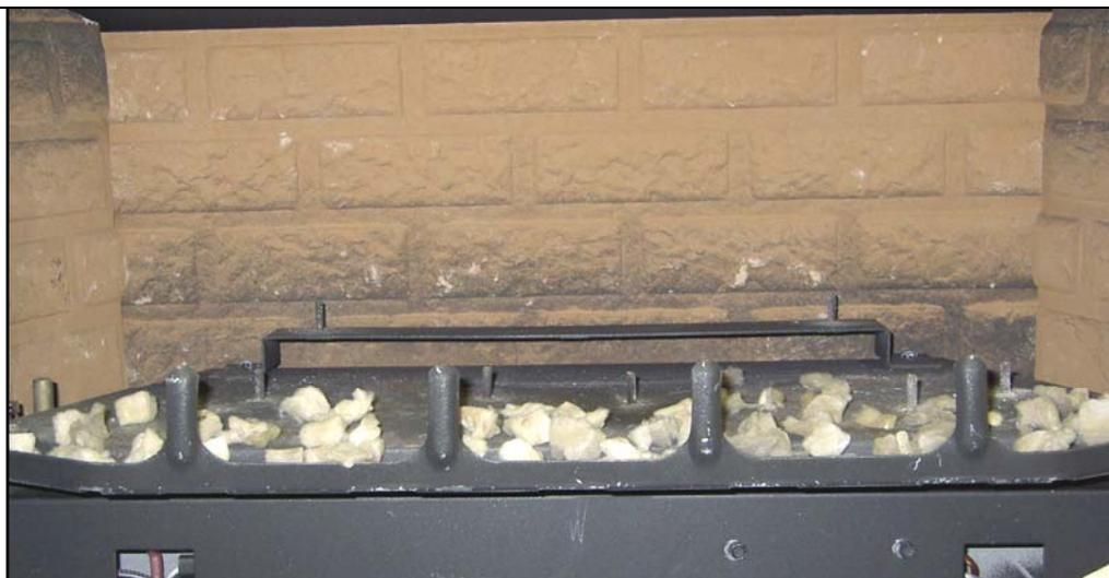
**WARNING :** Do not place the embers directly on the burner ports. A fire, explosion or excessive carbon monoxide (CO) may result, causing property damage, personal injury or loss of life. **Do not add more or different materials to the burner than the amount and type supplied with the unit.**
