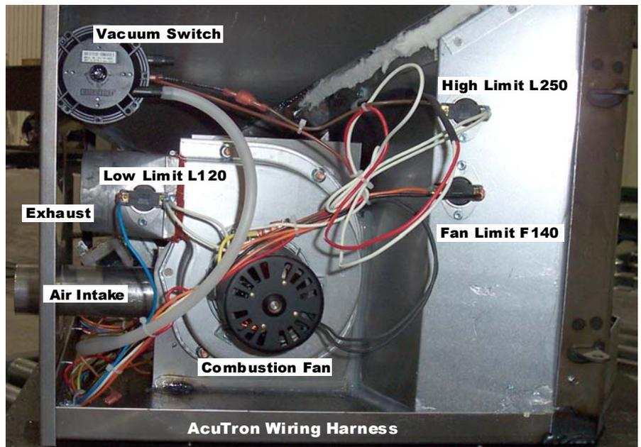
**If the power does go out, the pellet appliance will stop running. When the power comes back on, the stove will not restart if the switch is in the manual mode. If the exhaust temperature is above 120deg F or the switch is in the manual position, the stove will start to feed pellets again and may re-light itself.**
