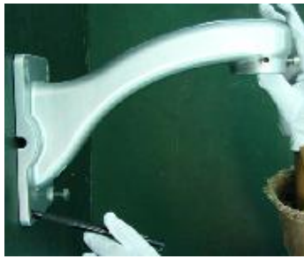
Figure 3-4 Determine position of screw installation hole
