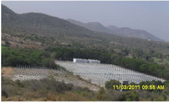
Fig. 1. Photograph of MST radar antenna array, transmitters rooms bird's eye view.
