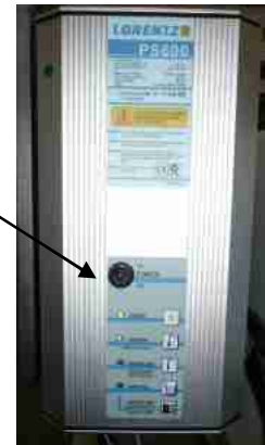
Emergency Dis- connect Switch
