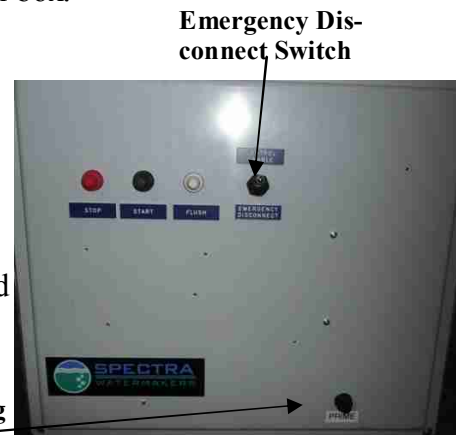
Boost Pump Priming Button
