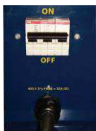
32 A D-curve circuit breaker
