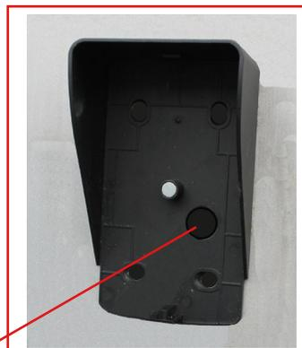
2. Mark a hole for the power and ethernet cable to run through. Remove the bracket, and then drill the holes. We recommend any holes you drill in your walls are sealed water tight after your cables are thread through.
