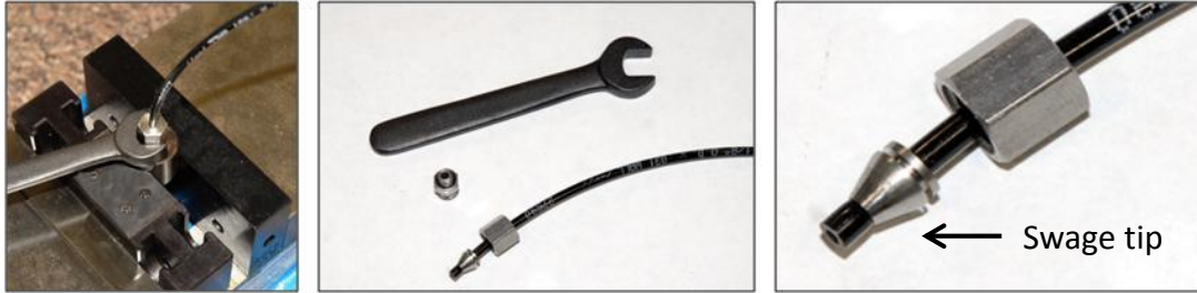
Figure 5. Swaging of assembled fitting by tightening in the pre-swage tool (left) and final swaged fitting on coolant line (right).
