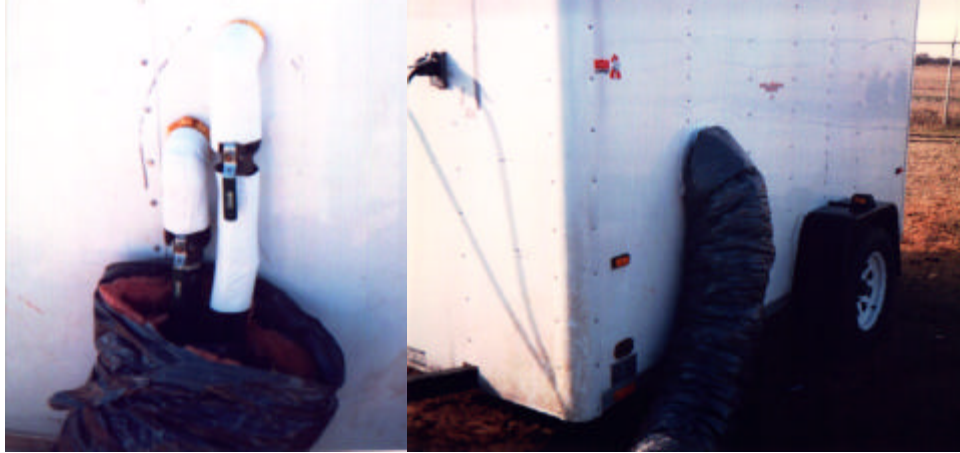
Figure 2-14. Exterior Insulation Connecting to the Trailer
