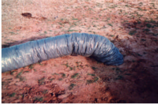
Figure 2-15. Round Duct Insulation Covering Pipe
