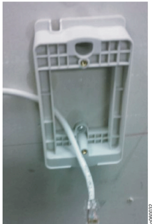
Figure 15: Pull the Category 5 Cable Through the Wall Bracket
