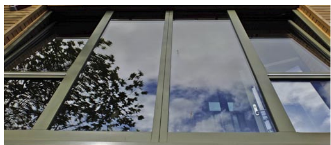
above: In hot weather the first floor glazing can be left on permanent vent and the outer set of ground floor doors can be left in the open position.
