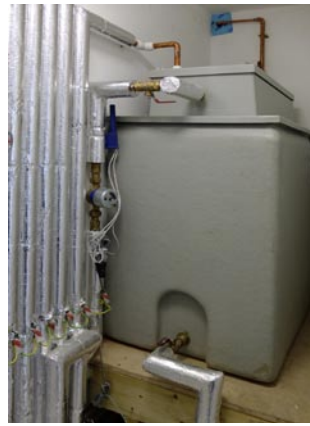
above left: The rainwater storage tank in the bathroom cupboard works on gravity and feeds the ground floor WC.
