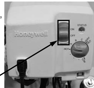
Gas control power switch
