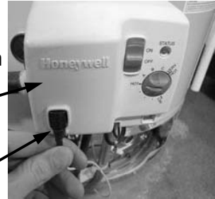
Spark igniter/flame sensor wire
