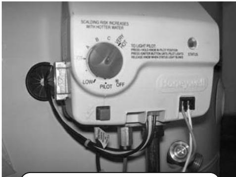
**Wire harness connected to the gas control**
