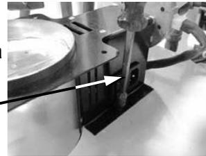
Step 7. Move the damper blade to the vertical position.
