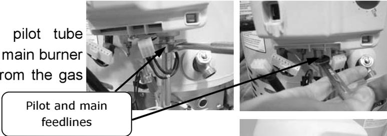
Step 7. Disconnect the spark igniter/flame sensor wire from gas control.
