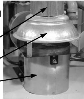
Step 4. Remove the draft hood from the damper and retain it for use on the new damper.
