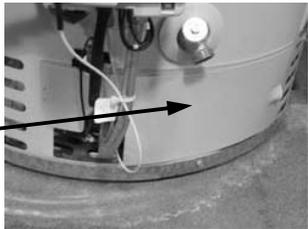
Step 5. Remove the (4) 1/4" hex drive screws holding the right side inner door in place.
