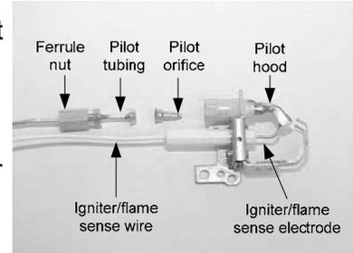
Step 16. Reassemble the pilot assembly and install it on the main feedline. Reinstall the burner assembly into the combustion chamber. Restore the gas supply and check for gas leaks.
