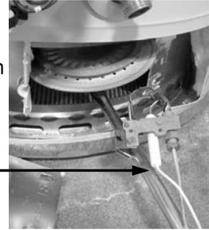
Step 9. Remove the pilot assembly from the main feedline using a 1/4" nut driver.
