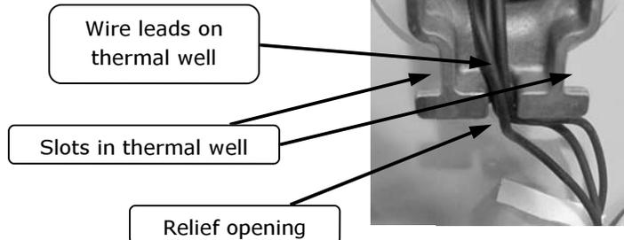
Step 3. Align the slots located on the thermal well flange with the tabs located on the back of the gas control.
