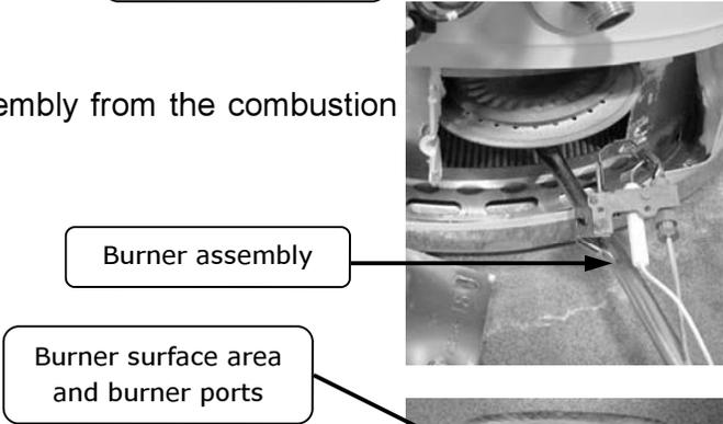
Step 9. Thoroughly inspect the burner surface area and burner port area and remove any loose debris.
