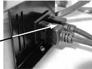
Step 6. Remove the two damper mounting screws using a 1/4" nut driver and retain for later use.
