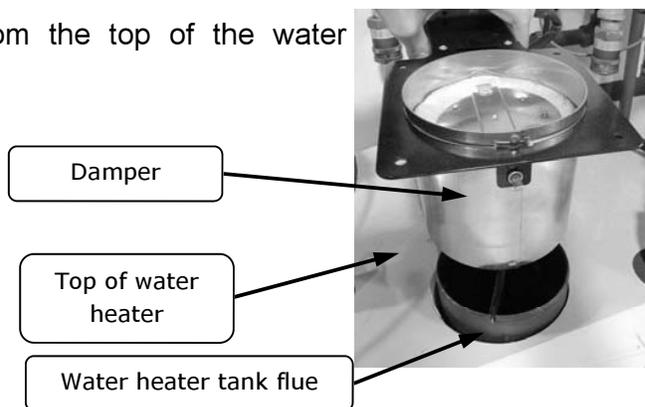
Step 7. Remove the flue baffle from the water heater.
