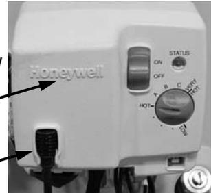
Step 6. Using the gas control service tool, p/n 239-45991-00, available from your BWC parts supplier, insert the tool into the back of the gas control.
