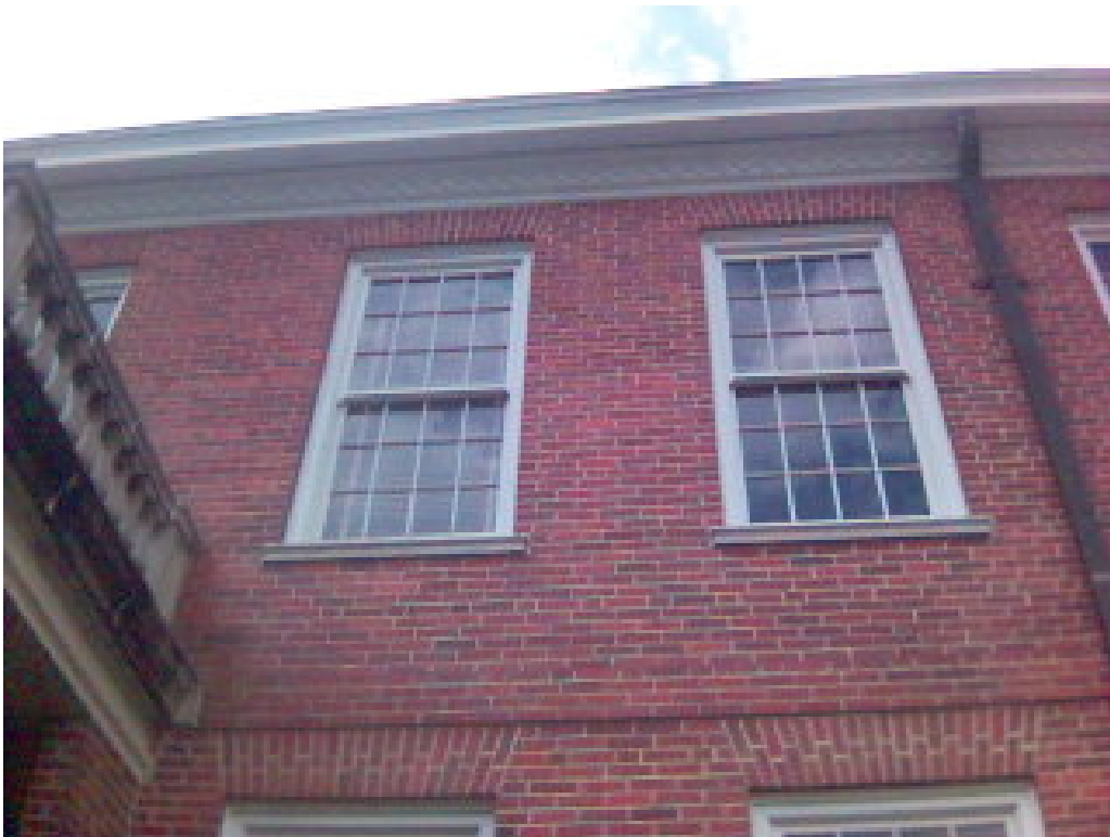
Figure 11.2 B Picture of the second story window where we threw out the box.
