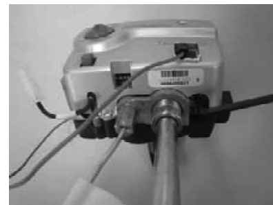
Gas Control shown in the "OFF" position
