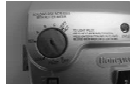
Gas Control shown in the "OFF" position
