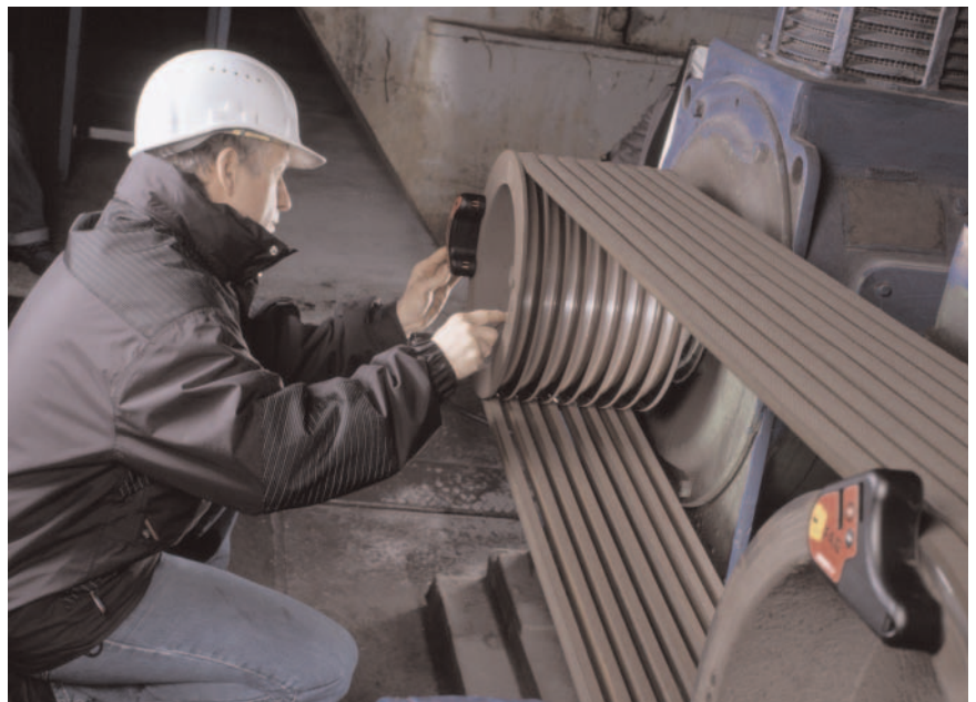
Alignment of belt pulleys
