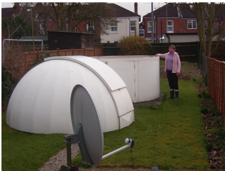
Fig. 3.7 Completed dome ready to mount on circular walls
