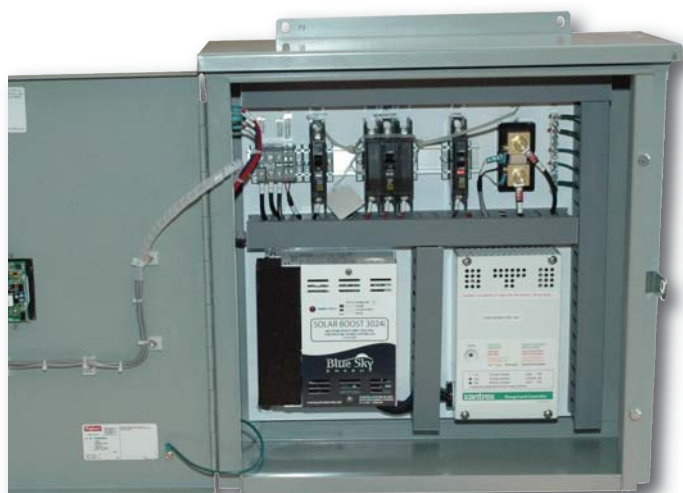
Figure 2-8 User Connection Wiring
