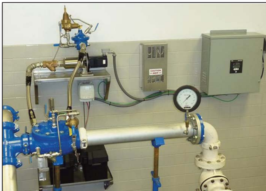
Fig. 1-2 X143HP Typical Application: Vault Installation
