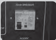
Fig.12 30mA leakage breaker Single phase off
