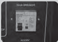
Fig.12 30mA leakage breaker Single phase off
