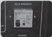
Fig.12 30mA leakage breaker Single phase off
