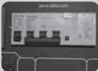
Fig.13 30mA leakage breaker Three phase off
