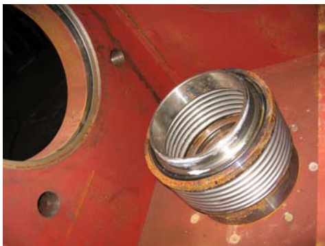
Figure 6-7 Suction flex adapter
