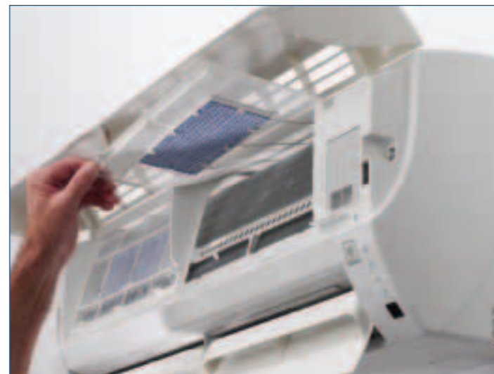
Air filters should be removed and vacuumed each week
