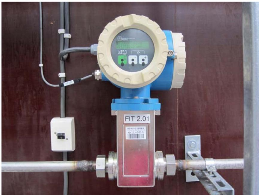
Figure 3.12: Water flow meter
