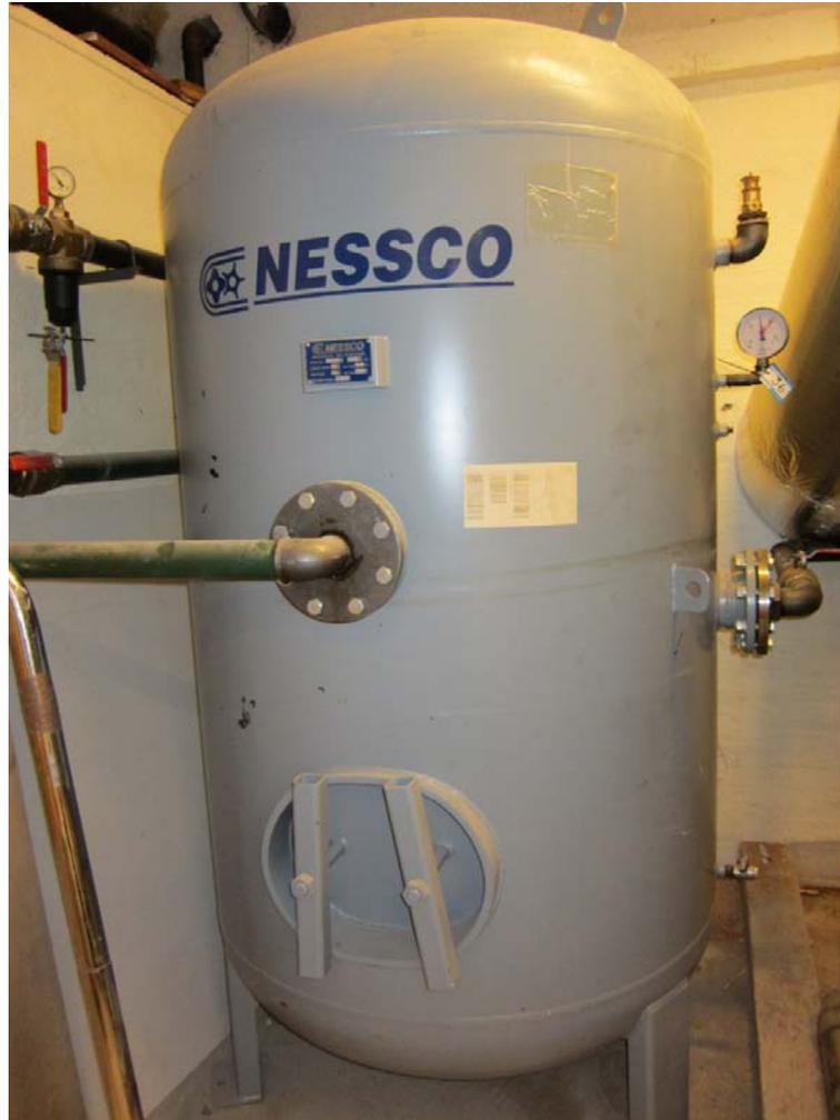
Figure 3.6: Air reservoir tank located in basement
