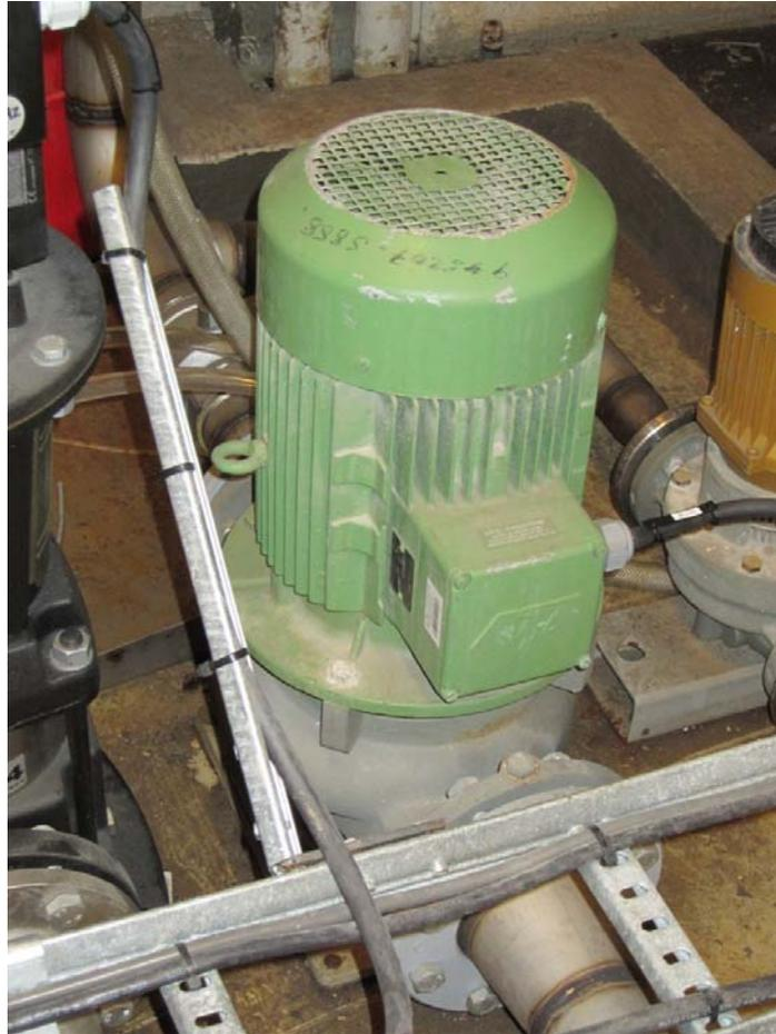
Figure 3.10: Centrifugal water pump
