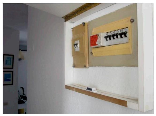
The picture shows the correct settings (all fuses are in the «up» position)
