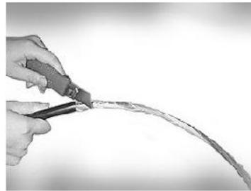
Remove plastic tape and dummy fillers. Clean the loose tube using jelly cleaner.
