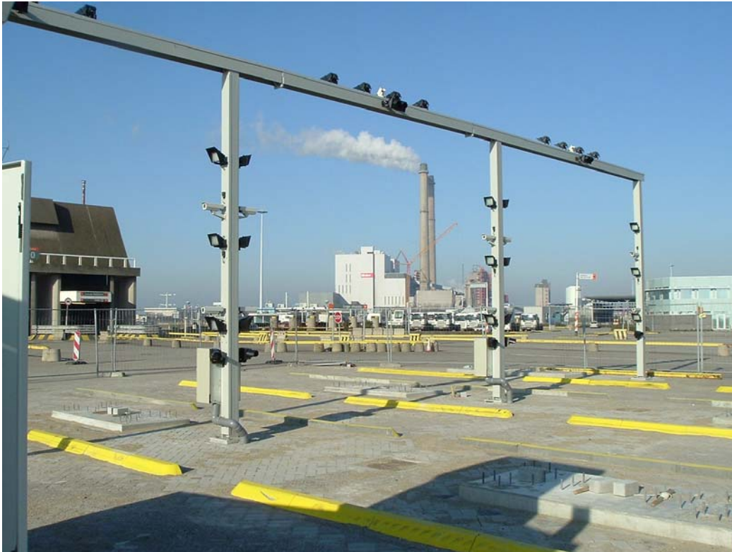
Photo 3.4.3: SeeGate2 Installation (Rotterdam, The Netherlands)
