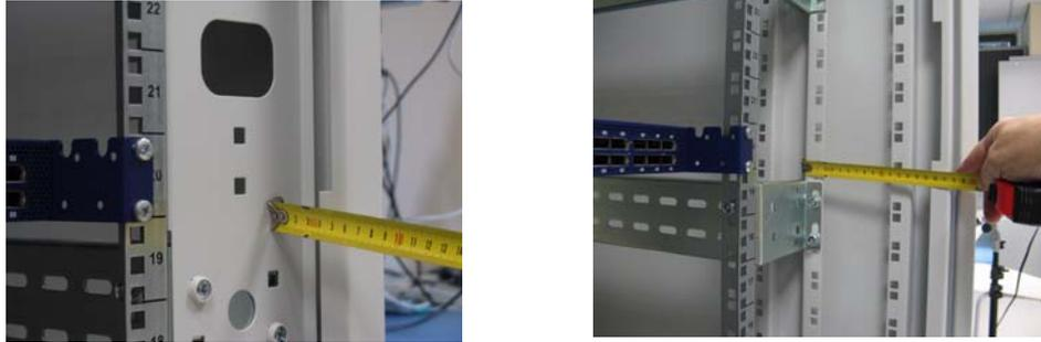
The distance between the rack and the door will be as little as 4 cm on one side of the rack and as much as 18 cm on the other side of the rack. Keep in mind that there can be as many as 36 cables connected to the switch.
