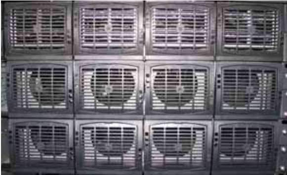
Safe solution. Blanks must be used to cover any open module slots.
