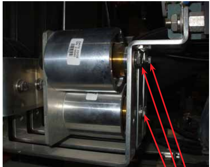
Bolts holding surge suppression assembly
