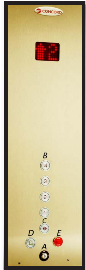
Figure 1 Cab Operating Panel
