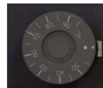
There is no need to switch the water heater off when it is not in use. The thermostat is fully automatic and only allows the gas control to open when the burner requires gas for heating. To adjust the thermostat settings refer to "[Temperature Control](#)" on page 35.
