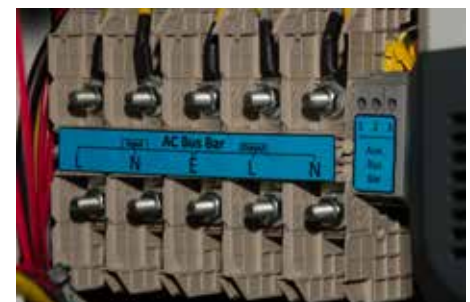
Fig. 6 - Bus Bar: AC In, AC Out & Auxiliary
