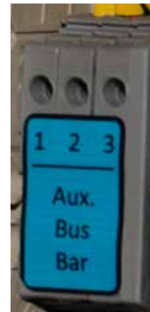
Fig. 10 - Auxiliary Bus Bar
